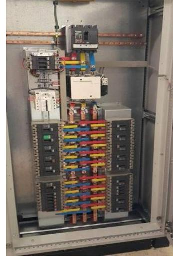
SMBD with Leakage Relay & Toroid
