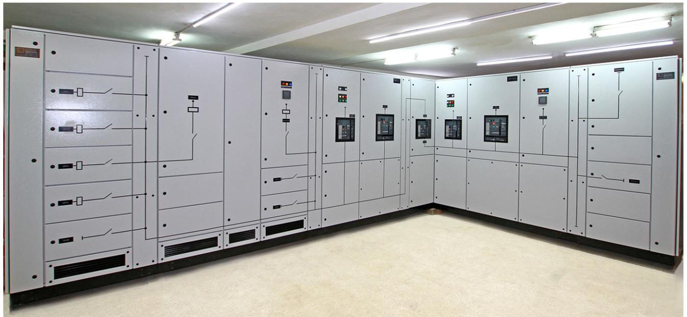
BUS-TIE 1600KVA With 2xATs-MDB, Between EDL & Synchronizing, Form-3B
